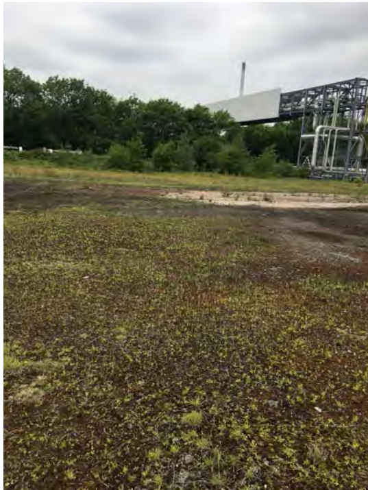
Photograph 11 | Former laydown area, including pipe bridge, looking south west.
